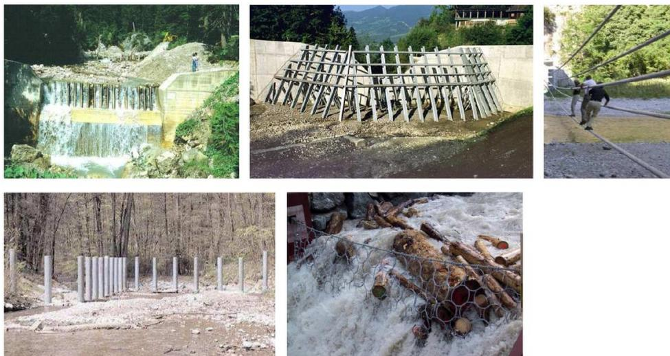
**Fig. 1** Images of different types of wood retention structures in the European Alps (higher centered and lower left images are from Lange and Bezzola, 2006; the lower right from Geobruigg, 2007).
